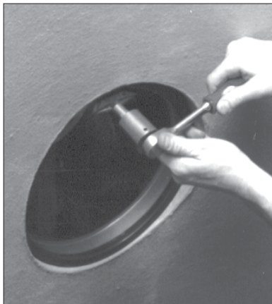
Install Kor-N-Seal I - Wedge Korbond with Socket Wrench & Torque Limiter
