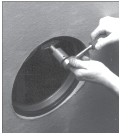
Install Kor-N-Seal I - Wedge Korband with Socket Wrench & Torque Limiter
