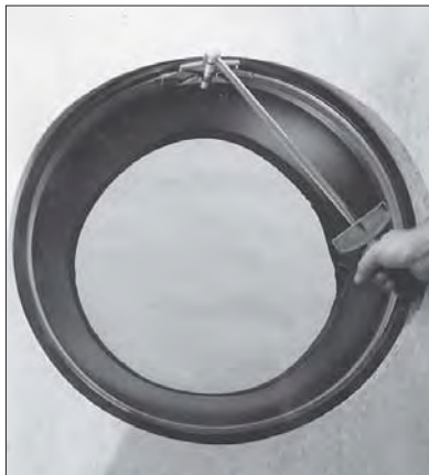
Install Kor-N-Seal II - Wedge Korbond with Standard Torque Wrench
