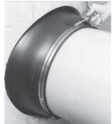
Install Pipe Clamp(s) with T-Handle Torque Wrench
