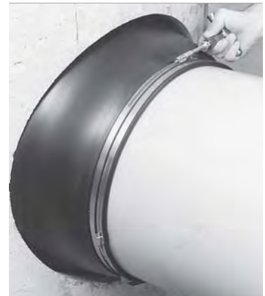
Install Pipe Clamp(s) with T-Handle Torque Wrench
